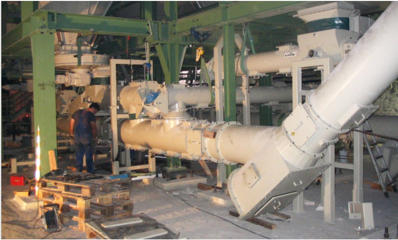
Erection of weighing-, filling- and inclining screw
